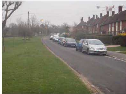
Photo 2.3 Shakespeare Road Between Burns Crescent & Scott Road
