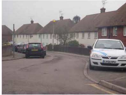
Photo 2.25 Burns Crescent View west from College Avenue
